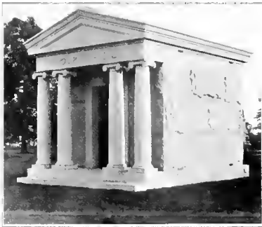
Number 9002. Erected in Mountain Grove Cemetery, Bridgeport, Conn., for D. W. and Carrie C. Thompson. It contains eight catacombs.
